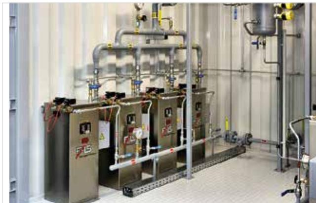
**LPG-Air-Mixing****unit FAS 4000****(Vaporizer + Mixing unit)**
